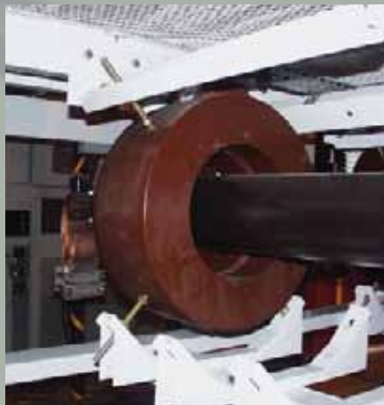
› ABG-24 Current transformer for generator designed to work with very high primary currents.
